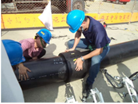
Connection of fire fighting pipes
