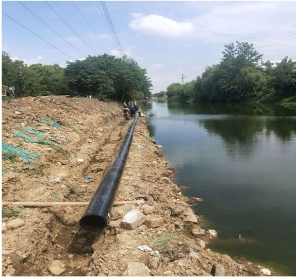
Pipe laying near river
