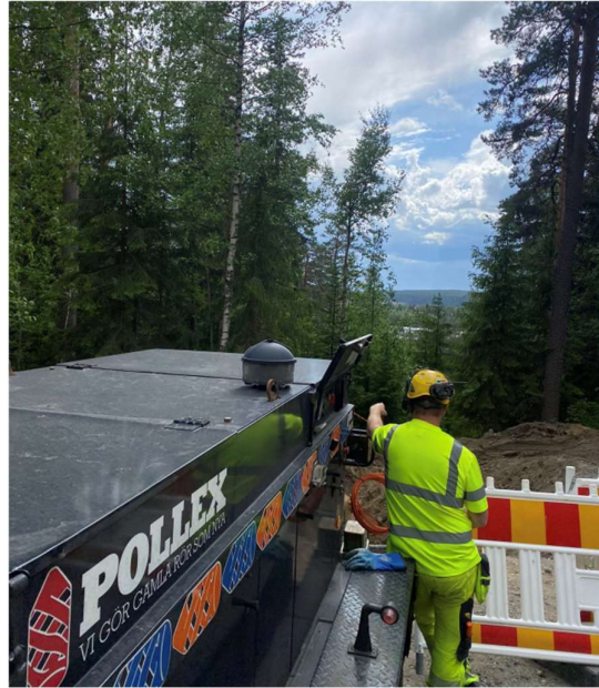
Fig. 9. The winch unit that pulled through the pipe liner
