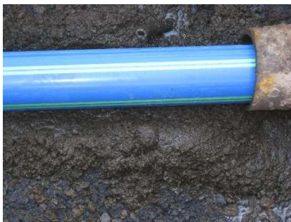
Relining of steel pipe
